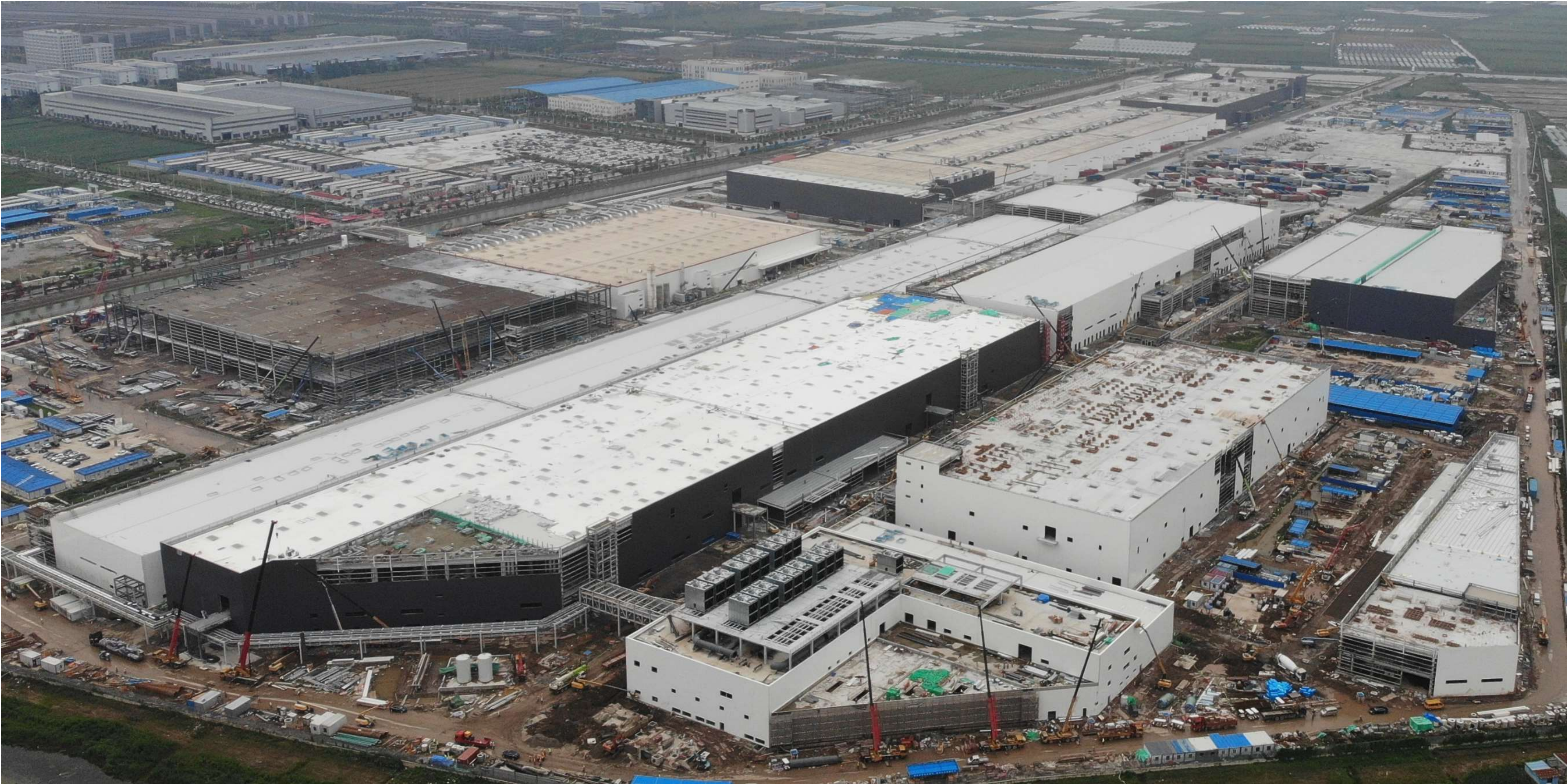
GIGAFACTORY SHANGHAI - MODEL Y FACTORY (FOREGROUND); MODEL 3 FACTORY (BACKGROUND)
