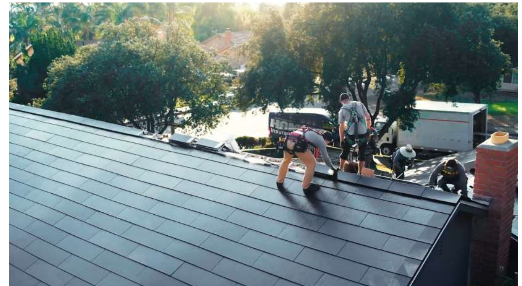
Solarglass Roof installation
