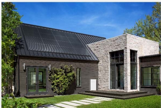
Powerwall with retrofit solar
